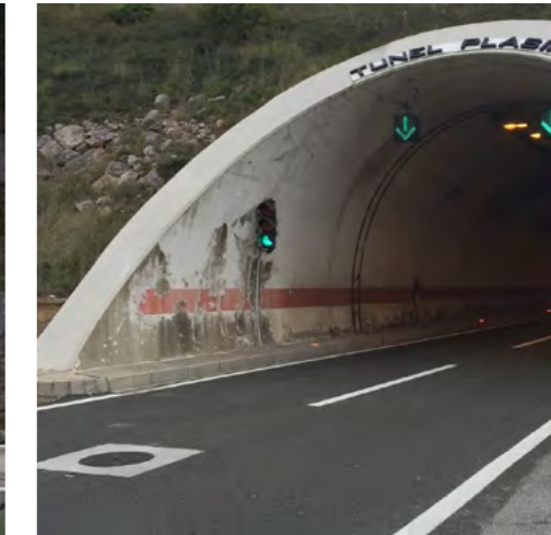
HAC A1 Tunnel Grič, Plasina, Croatia
