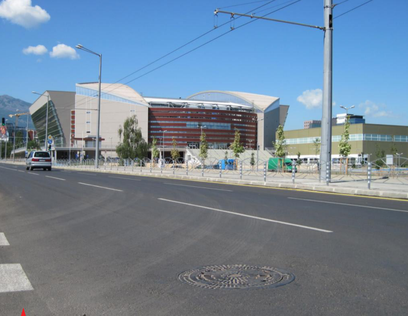
ACO Multitop - manhole covers in the reconstructed road
